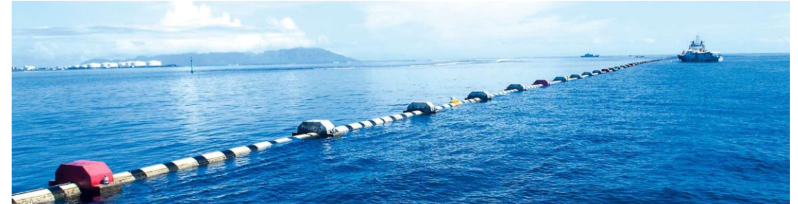
A pipe measuring nearly 4 kilometers in length cools the capital's new hospital using seawater.
